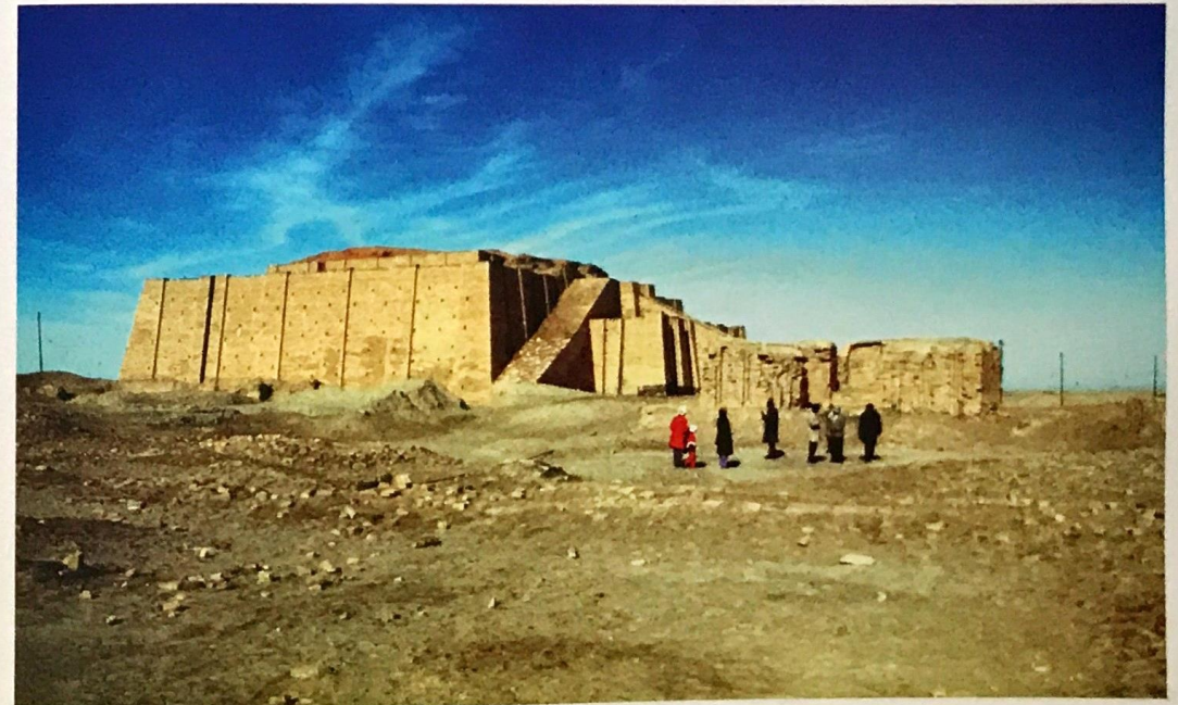
Iraqis have partly rebuilt the solid mud-brick ziggurat at Ur with long outside staircases and massive walls. The original upper stories and the small shrine at the top are missing.
