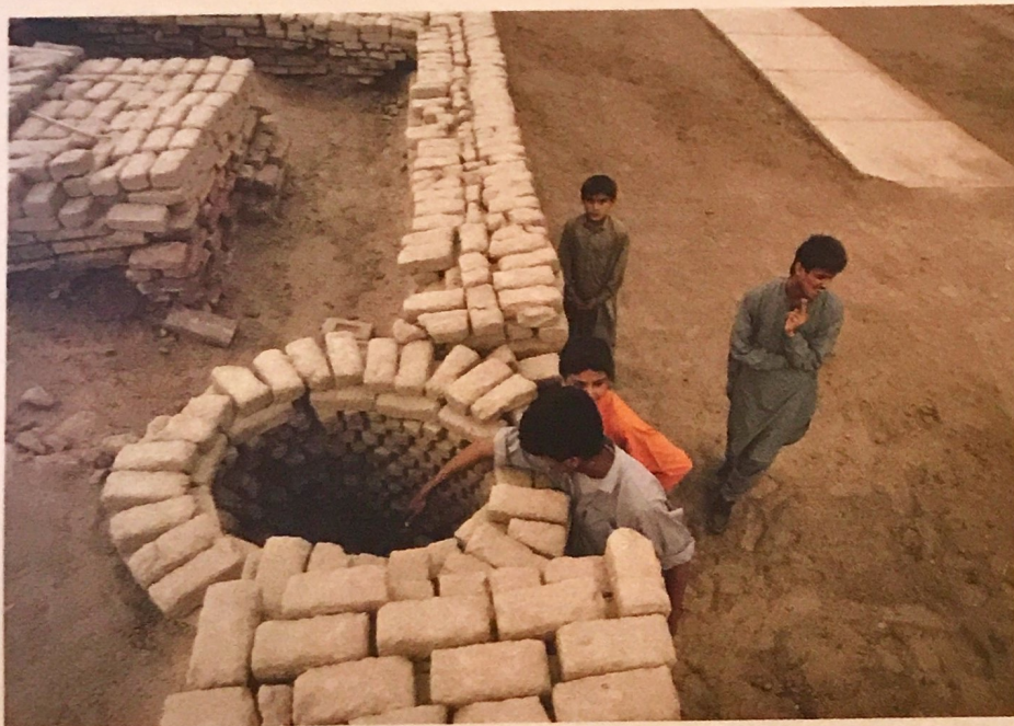
“ ” Public well and bathing platforms, Harappa, about 2500 BCE
